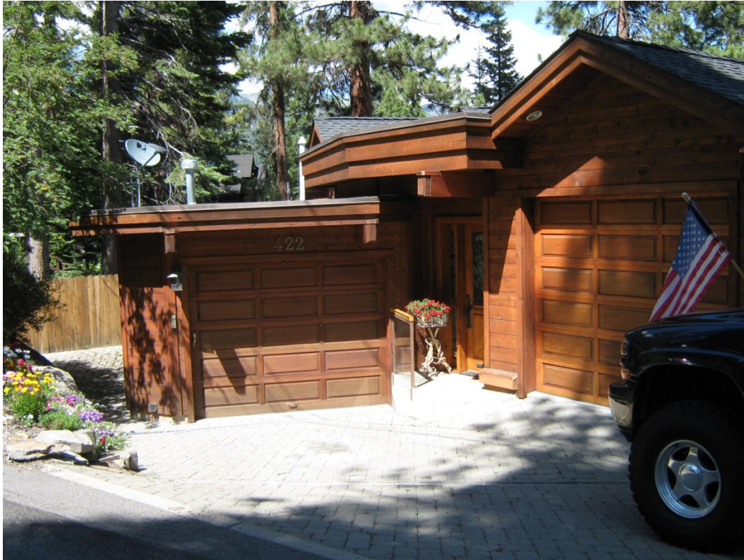
Adjacent property (422 Gonowabie): VA4-31-96 reduced the front yard setback to zero.
