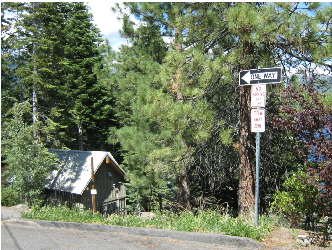
Gonowabie is a one way street due to its narrowness. Despite the no parking sign, residents park in the street ROW where possible because of a general lack of parking. The road was never accepted for dedication but the county maintains it anyway.
